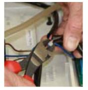
**5** Using Wire Clippers (or a sharp knife) carefully cut and remove the cable tie securing the power leads between the two halves of the unit.
